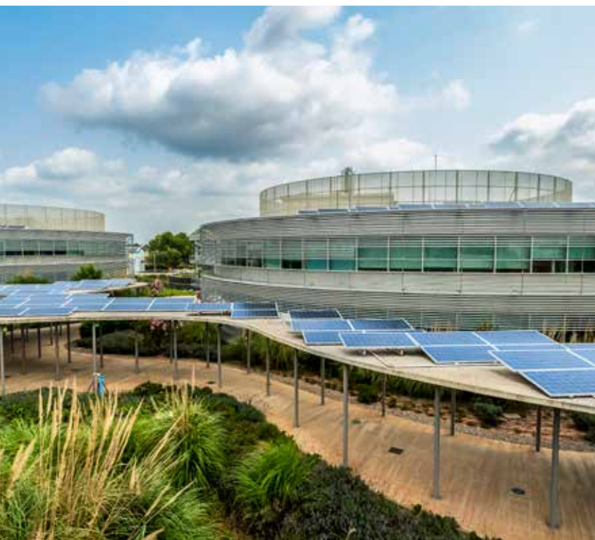
PV Panels at UNGSC in Valencia. UN Photo/Luca Nestola.
