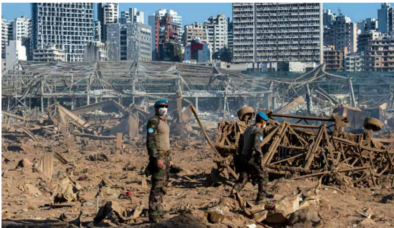
Port of Beirut, following the 2020 explosion. UN Photo/Pascual Gorriz.
