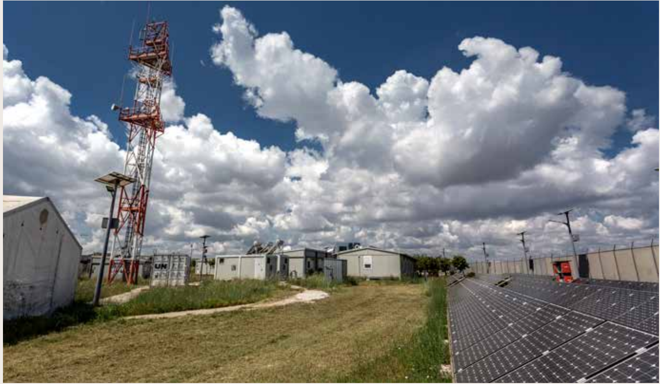
The Green Island was designed to simulate a 30-person camp in the field. It features UNGSC's crosscutting capabilities, for example, renewable energy installations, prefabricated structures, and communications modules that are part of the strategic deployment stocks for rapid deployment, as well as sensors for real-time data collection. Designed by UNGSC engineers and built by our mission support team, the Green Island provides a real-life testing, integration, and training ground. Photos by Alejandro Vicuña Leyton.
